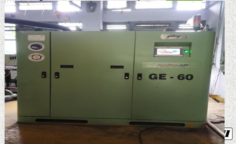
Use of Baby Compressors for individual shop in place of centralized compressed air <u>piping system</u>
